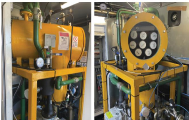
Vacuum Chamber for Gas & Water Removal
