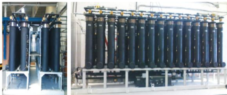
Polishing Module, 30 Columns 5400 kg TURBOSORB
